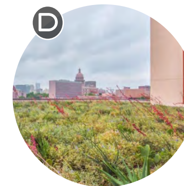
D GREEN ROOF on top of the building on Flex Area 4, the Revival tract
